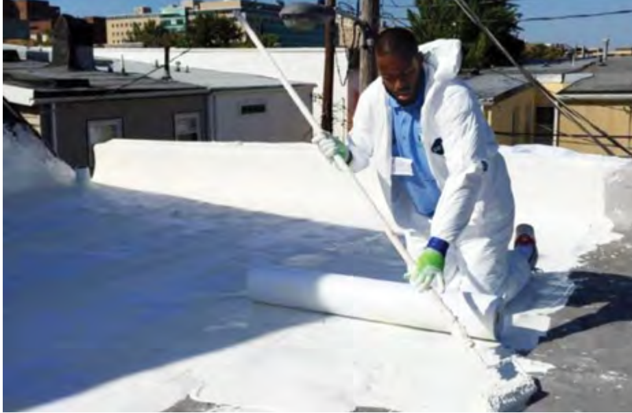
Exhibit 8. Cool roof installation at the Resiliency Hubs pilot.
